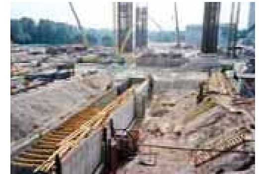
Bau Ofen 11 – September 1994
